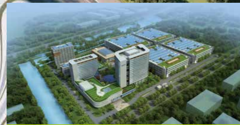
汇川联合动力有限公司办公大楼 Office building of Inovance Automotive
